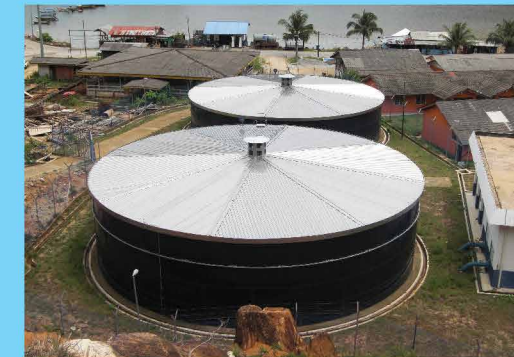
Stainless Steel Roof Pulau Redang
