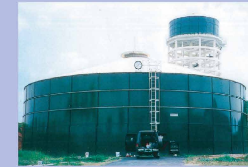
1996 Golf Resort-220,000 gallons (Elev.) & 750,000 gallons (Ground)
