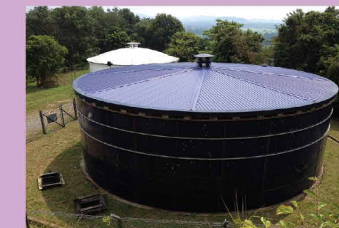
Kg. Jenalik, Kedah. Bulid 1990 Service & Roof Replacement-2011
