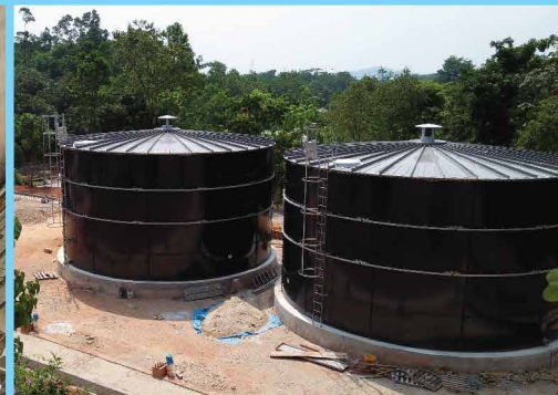
GRP Roof Perak
