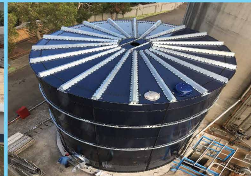
Tapped Beam Roof Taiwan
