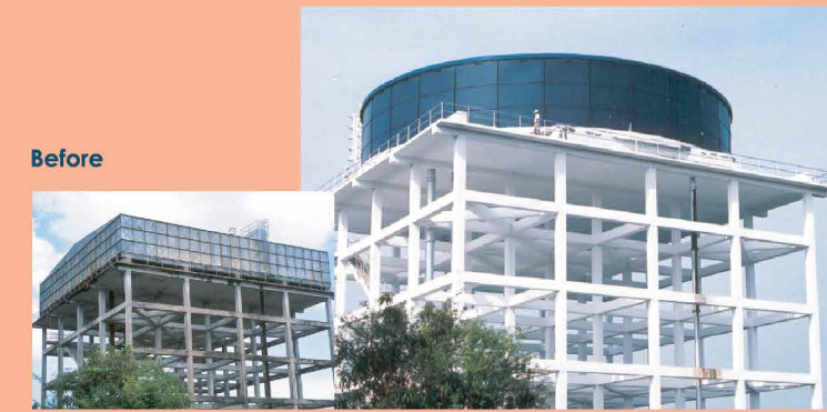
Before Press Steel 500,000 gallons After
