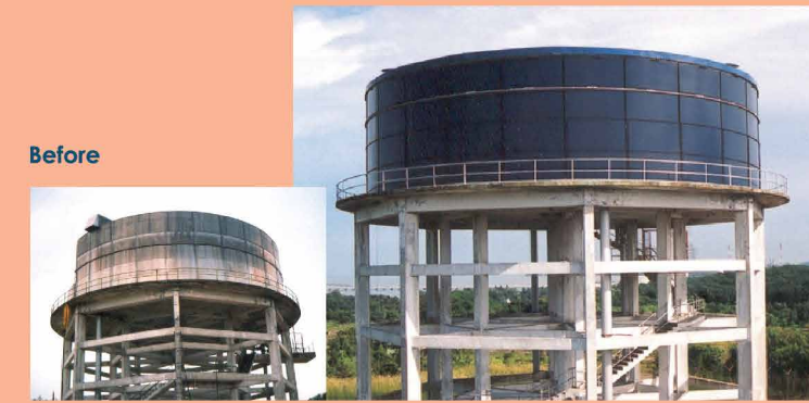
Before Liner Tank 400,000 gallons After
