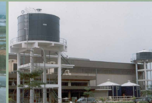
1994 5th new tank built next to existing tanks
