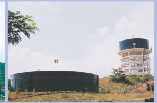
2001 2nd set installed-250,000 gallons (Elev.) & 600,000 gallons (Ground)
